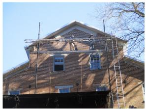
The frieze boards are wide flat planks laid against the brick wall directly under the eaves. They are intact on the front of the building, but had been missing for decades on the back. This work was accomplished in only two days, on January 26 – 27, 2023.
